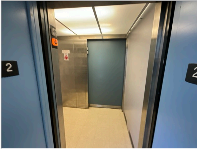
LOBBY LOOKING AT CABS
