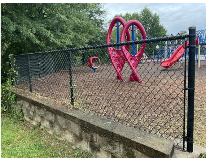
35 - RETAINING WALL, FENCING
