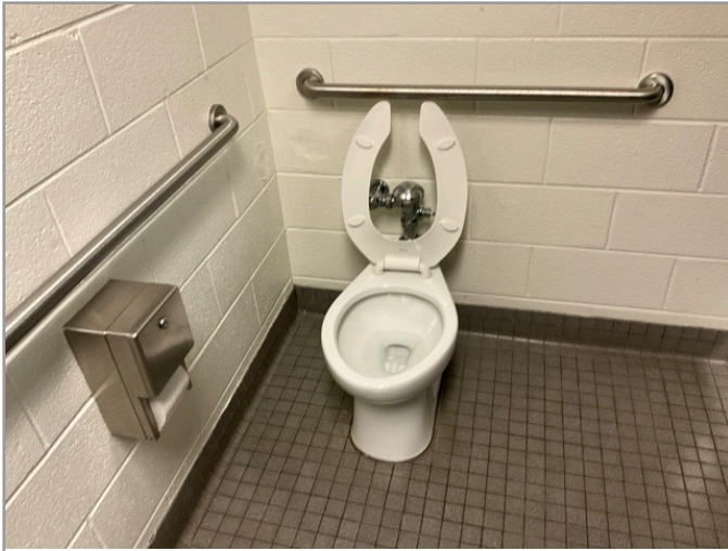
TOILET STALL OVERVIEW
